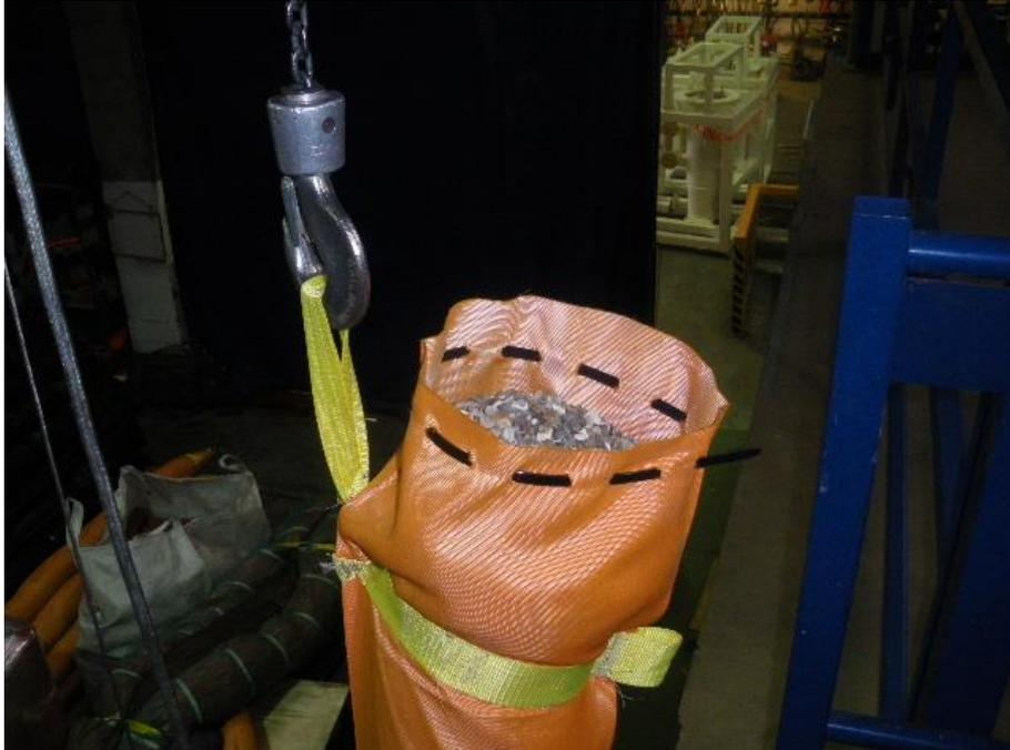
3) When the tube is adequately filled, seal the end using the attached string / tie wrap:
